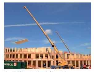
*Figure 7:* CLT panels being lifted into position – construction should be fast compared with most traditional methods, although additional resources may be needed in the planning and design stages (Courtesy of Kier Eastern)
