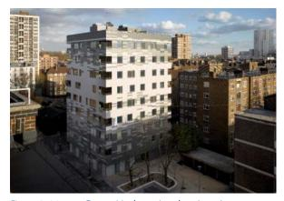
*Figure 2:* Murray Grove, Hackney, London, is a nine-storey block – CLT panels are used as loadbearing walls and floors (Courtesy of Will Pryce)
