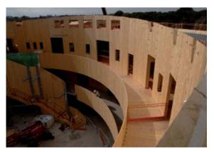
*Figure 6:* CLT forms solid loadbearing planes, just like masonry walls and concrete slabs, with offsite precut windows and doors (Courtesy of Kier Eastern)
